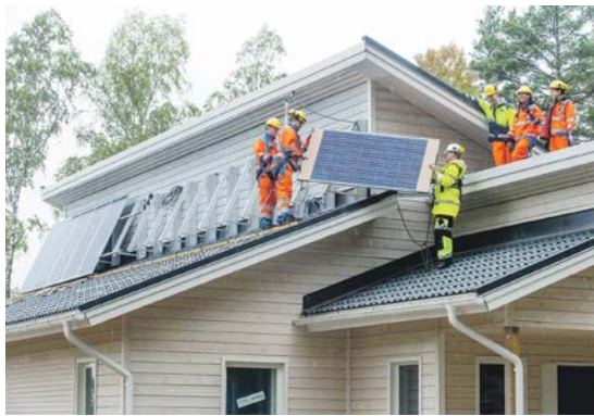
Solar panel installation
